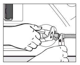
■ Using two wrenches tighten the flexible gas line connection.
